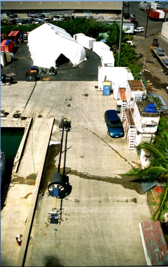
Snug Harbor Facility
